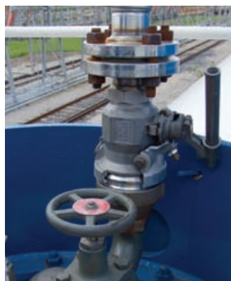
TPC has upgraded its railcars that transport butadiene to the OPW Engineered Systems’ Drylok™ coupler.
